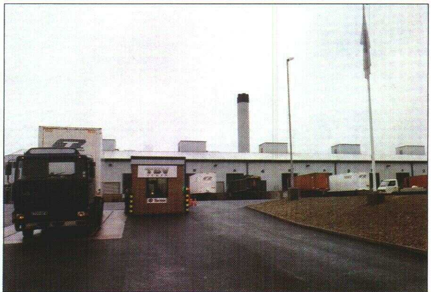
The West Midlands Whole-Tyres-to-Electricity Facility at Wolverhampton, owned and operated by Elm Energy and Recycling (UK) Ltd, was the first power station of its kind in the UK. It generates over 175 000MW of electricity per year for the Grid by burning used whole tyres, and also produces useful by-products for the steel and zinc industries. Elm Energy's initial proposal for a tyre combustion facility was made in 1989, in response to the Department of Trade and Industry's requirement for a long-term solution to the nationwide problem of scrap tyre disposal.
